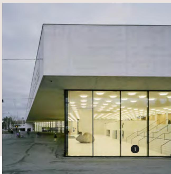
**1. Fassadengläser:** TG-ESG®-H 10 mm 50/22 II, 16 mm CU SZR, TG-ESG®-H 8 mm ONE II, 16 mm CU SZR, TG-ESG®-H 10 mm von SAINT-GOBAIN.
